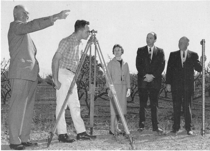
In March 1963, college district trustees observed the topographical survey of what was to become the site of De Anza College. From left are Hugh Jackson, president, Foothill Junior College District Board of Trustees; Hank Young of Mackay and Soms, an engineering firm; Mary Lou Zoglin, trustee; Dr. Robert C. Smithwick, board clerk (now CHCF board member); and A. P. Christiansen, trustee. Photo from Foothill-De Anza District Archives.
